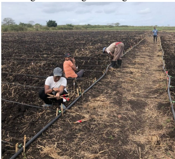
Figure 2: Fixing irrigation pipes
